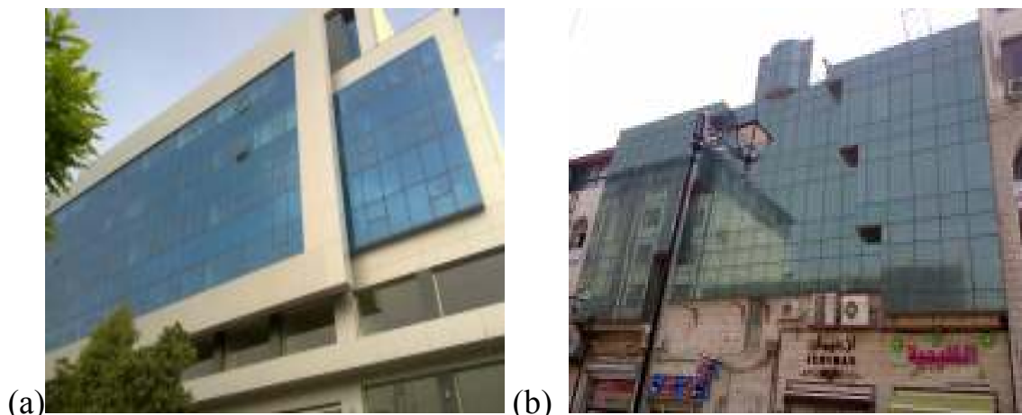
Figure (66): The use of glass curtain wall – Ramallah. Photo by: the author, 2011
