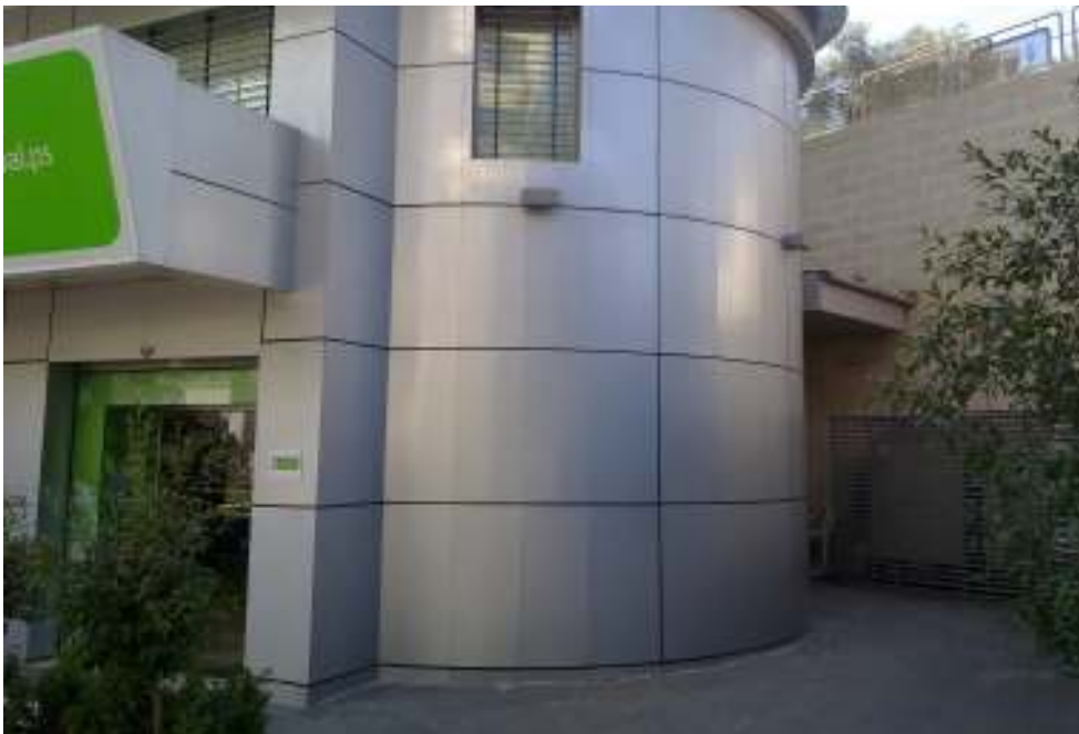
Figure (59): The use of Alucobond for wall cladding in Jawwal Exhibition in Nablus.
