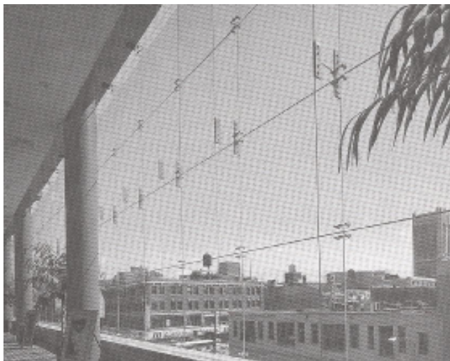
Figure (70): Bended glazing curtain walls
