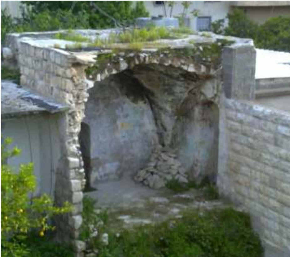
Figure (10): Demolished small structures in Nablus where the cross vault roofing system is clear
