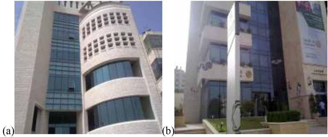
Figure (64): Glass curtain wall Bank of Jordan building – Ramallah. Photo by: the author, 2011.
