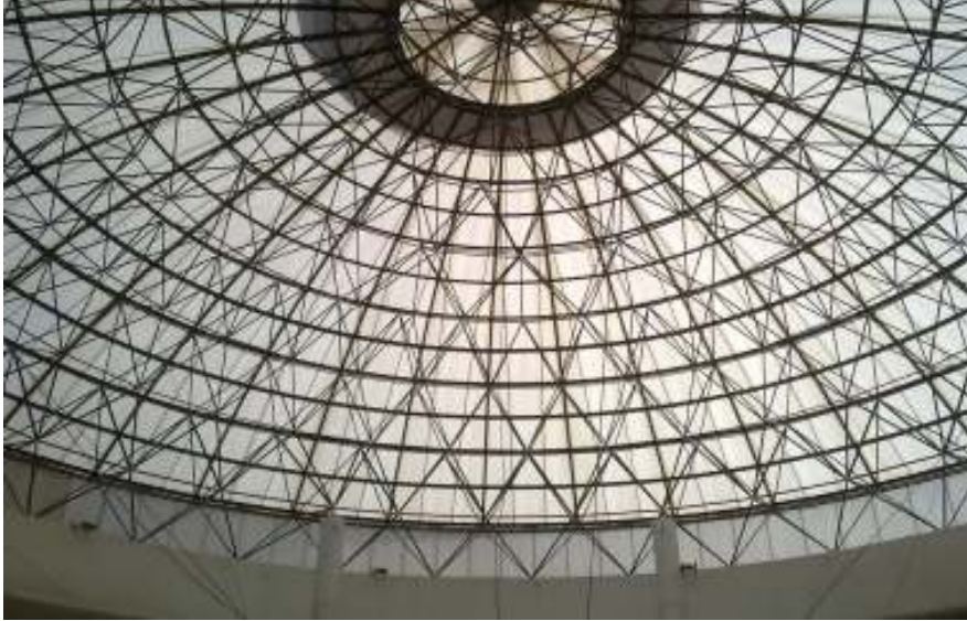
Figure (35): Space frame dome at Nablus commercial center. (A view showing the court yard roof)
