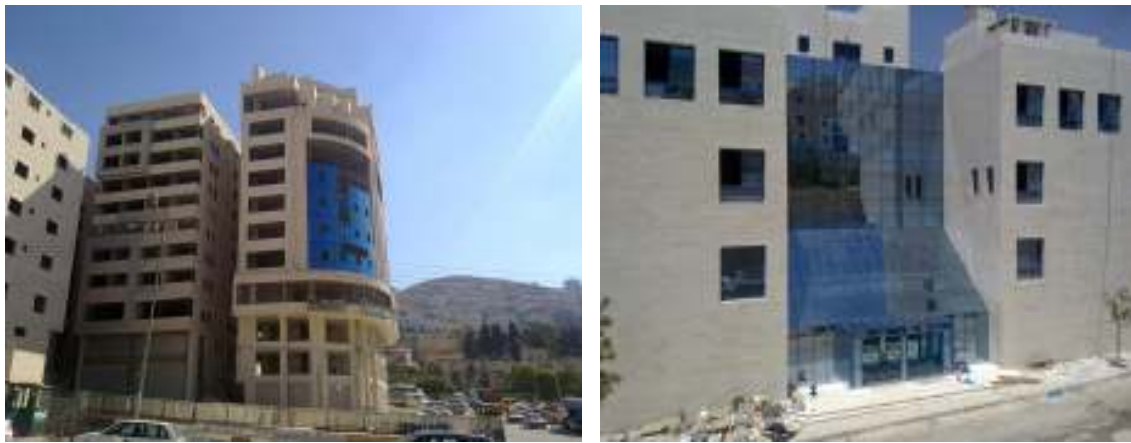
Figure (65): The use of glass curtain – Nablus. Photo by: the author, 2011.
