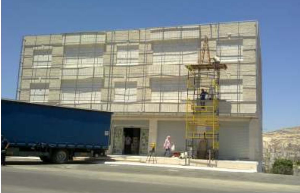
Figure (60): The use of metal plates for wall cladding in Sbeitany Exhibition in Nablus.
