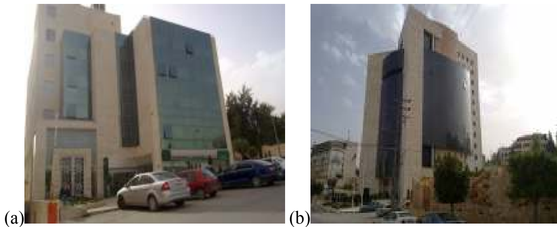
Figure (63): The use of glass curtain walls – Ramallah. Photo by: the author, 2011.
