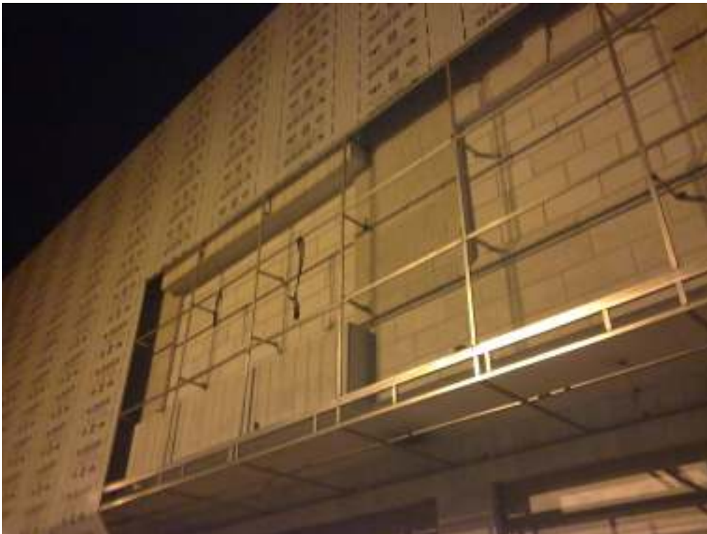
Figure (61): The use of metal plates for wall cladding in Sbeitany exhibition in Nablus-cladding face.
