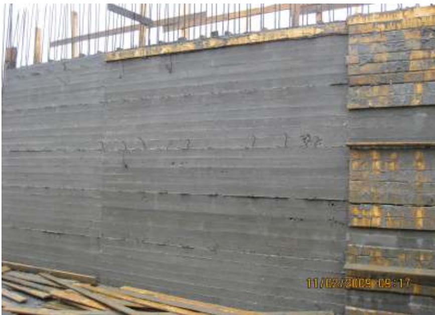
Figure (41): A photo shows a concrete wall.
